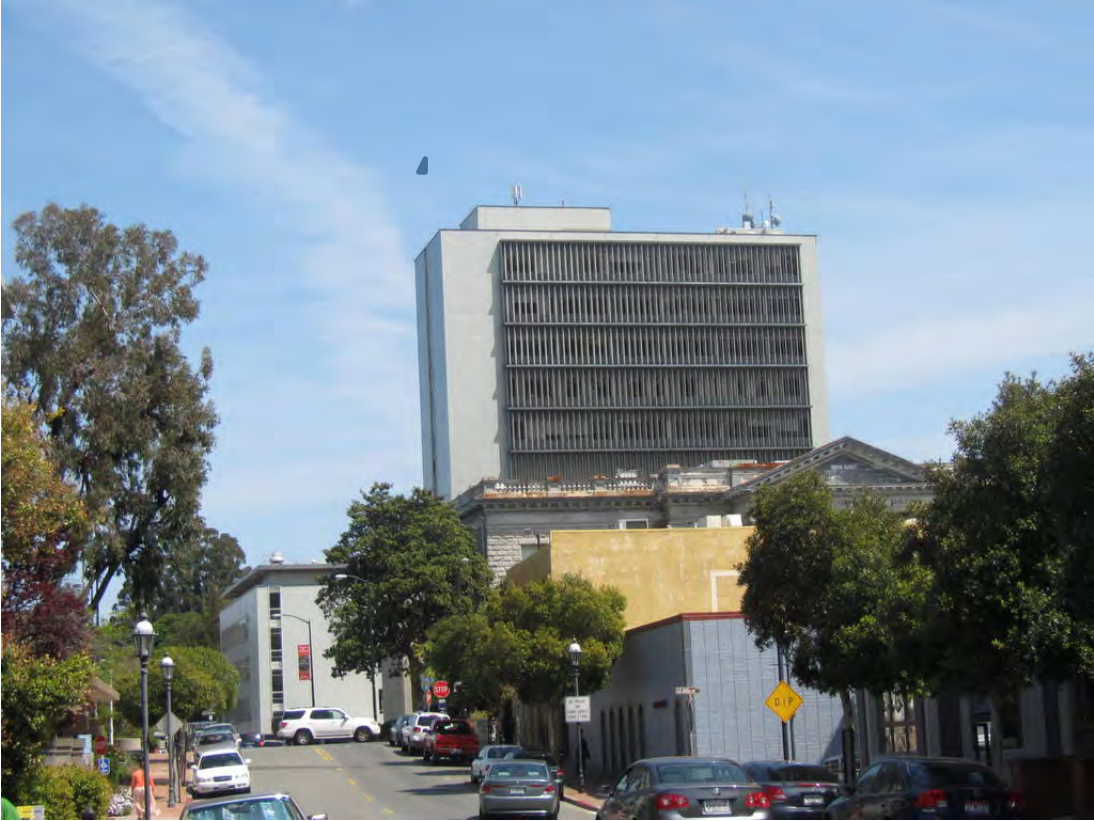
LTE Antennas at 651 Pine Street
